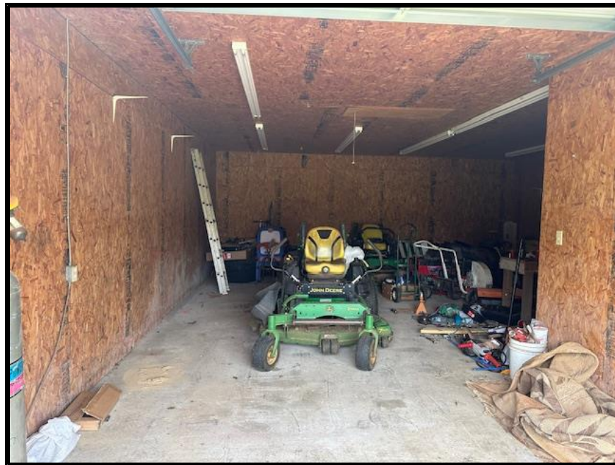
Interior of Shop Building
