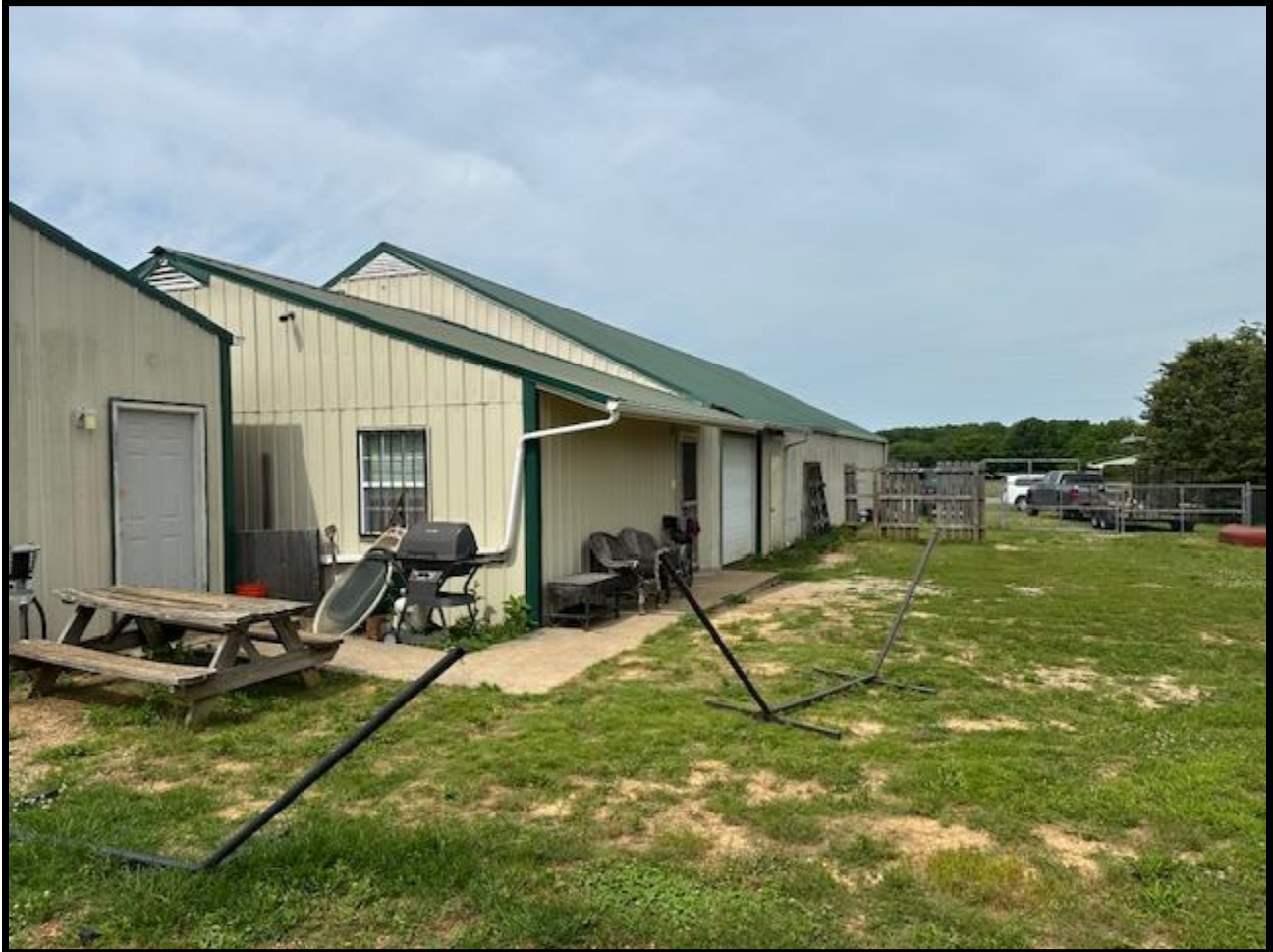
Rear View Looking West
